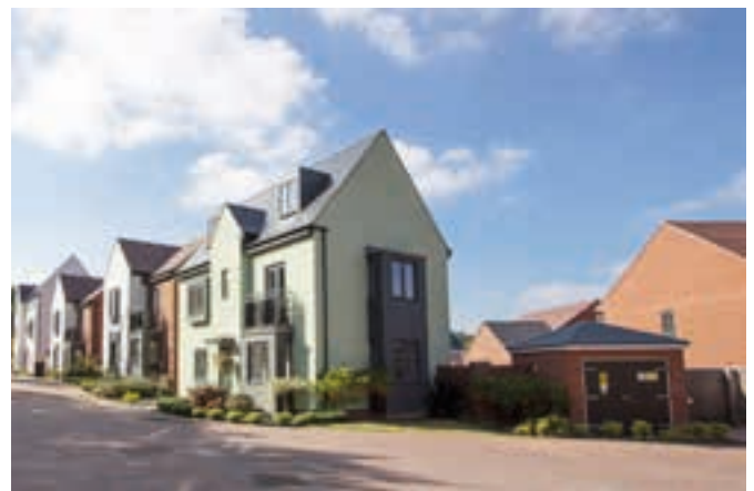
Precedent photograph illustrating integration of substations with material palettes to match neighbouring built form.
